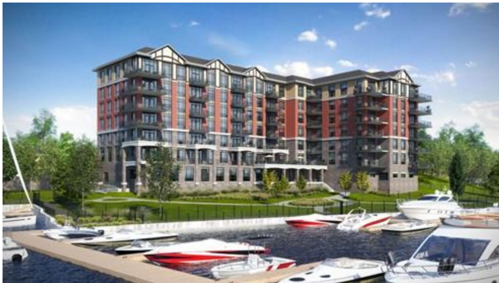
Stone & South on the River Gananoque, ON
